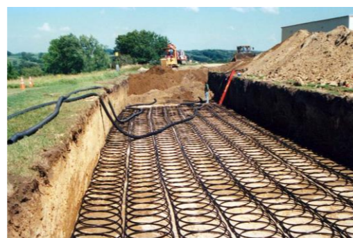
Figure 47 – GSHP coils
