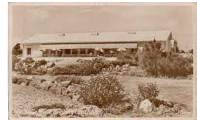
Figure 14 – Rock Garden Pavilion (Google Images)
