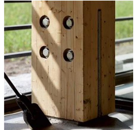
Figure 84 – Steel Knife Plate
