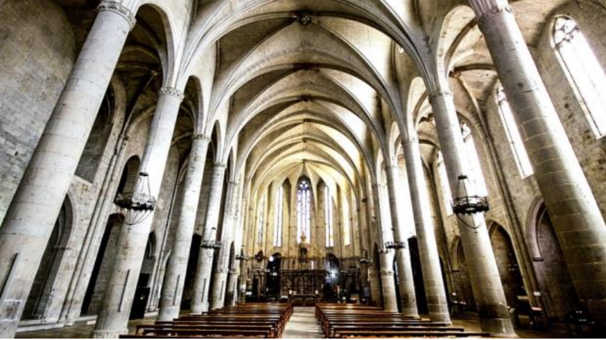
Figure 22 – Typical Cathedral Columns
